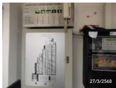
Graphic Annunciator Fire Alarm System
