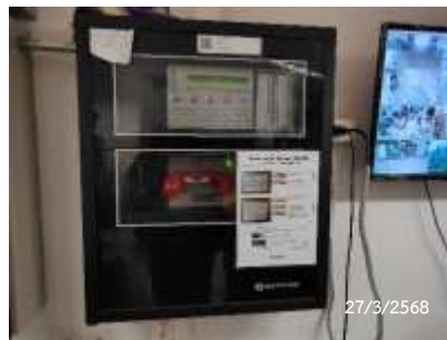
Fire Alarm Control Panel
